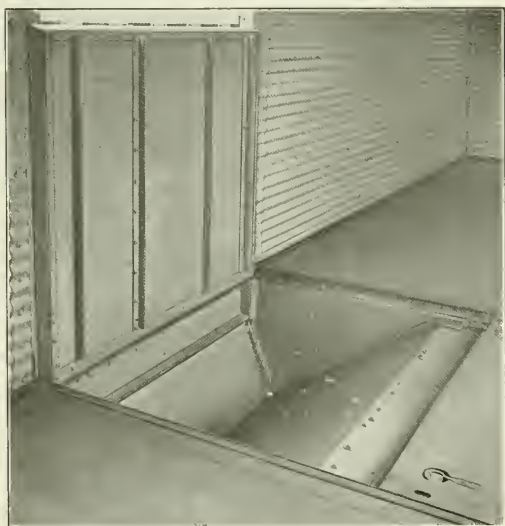
Hopper Bottom in Connection with Metal Sheathing.
